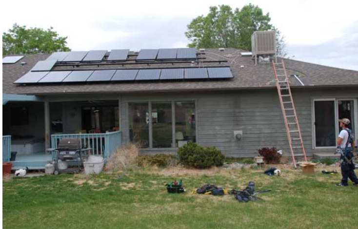
Nearing the end of day one of installation
