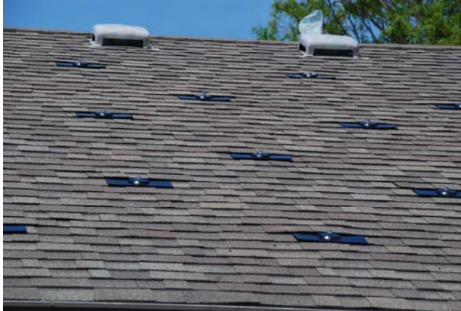
'Feet' are the first thing they attach to the roof
