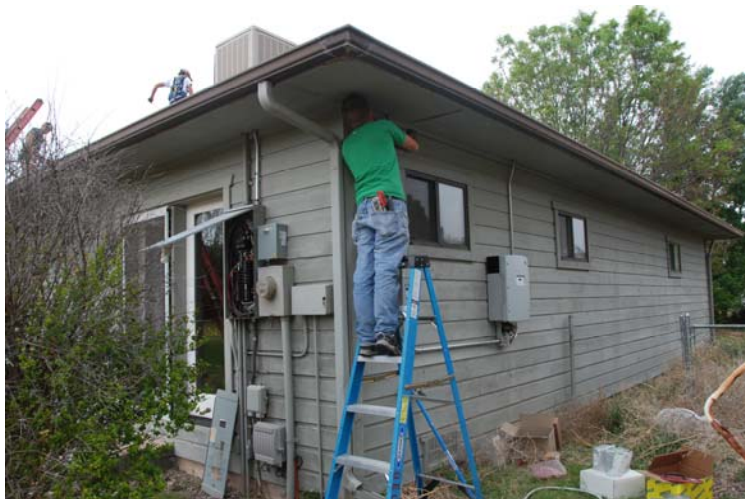
A certified electrician installs the electric control box)
