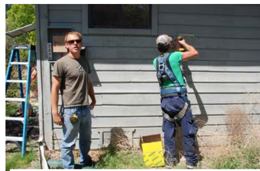
Finding a location and preparing for the electrical box.
