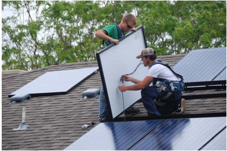
Connecting the electrical wires beneath the panels
