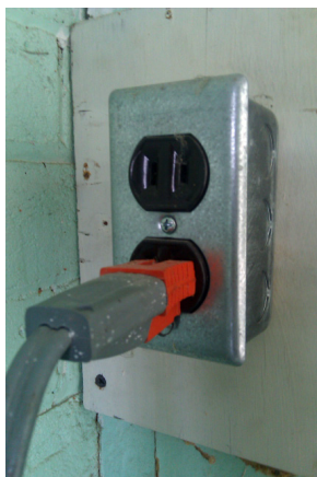
Figure 3. Some outlets require use of a 3-prong adapter to host a power monitor.
