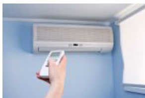
Air handler of a ductless mini-split. Source: Hobaica Services
