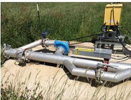
Figure 2: Irrigation water diverted to a turbine before being used to irrigate. Photo: Blake Osborn
