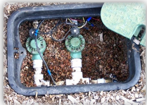
Figure 3. Valve box with two zone valves.
