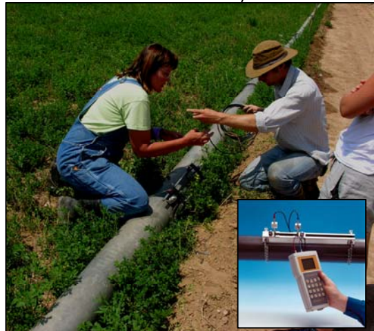
Figure 1 : Installing the Ultrasonic Flowmeter (notice sensor is at 45° to pipe center or “1:30” on a clock face)
