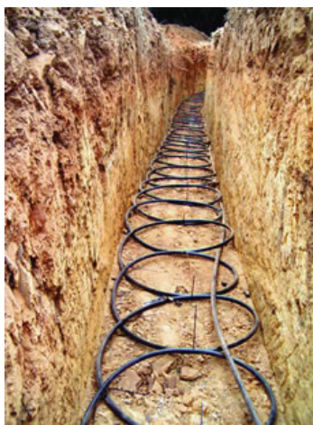
Horizontal loop field photo credit: Air Solutions
