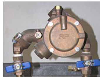
Figure 4: Reduced Pressure Device.
