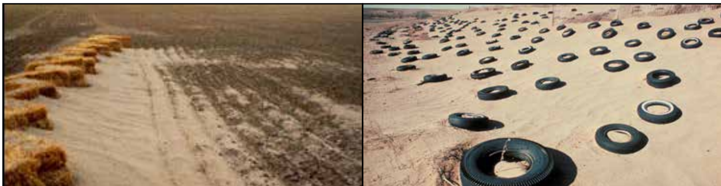
FIGURE 31. Artificial barriers such as hay bales (left) or objects to create roughness (right) are temporary controls.
