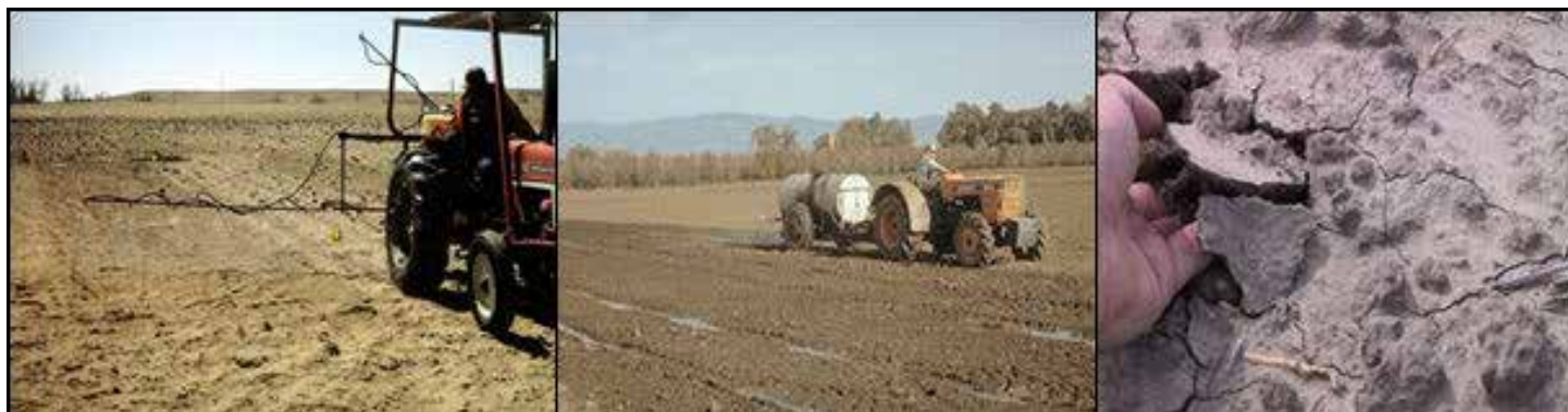
FIGURE 32. Soil stabilizers bind particles together to make them less erodible.
