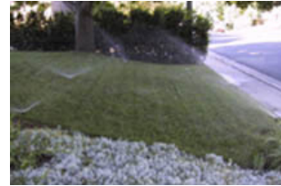
Figure 7: Line hardscape areas with heads to throw water back into the landscape, never within the landscape throwing water towards the hardscapes.
