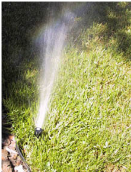
Figure 5: Rotor heads rotate slowly sending out one or more streams of water to cover areas larger than spray heads.
