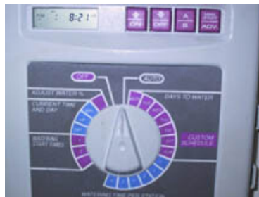
Figure 1: An irrigation controller with capability for changing water percentage for seasonal adjustment, and setting multiple start times for irrigation cycling.
