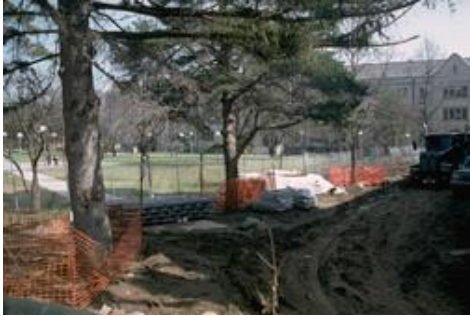
Figure 6: Construction vehicles can damage the existing soil structure by compressing soil particles.
