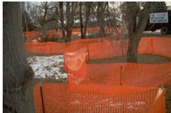
Figure 2: Highly visible tree protection barriers.
