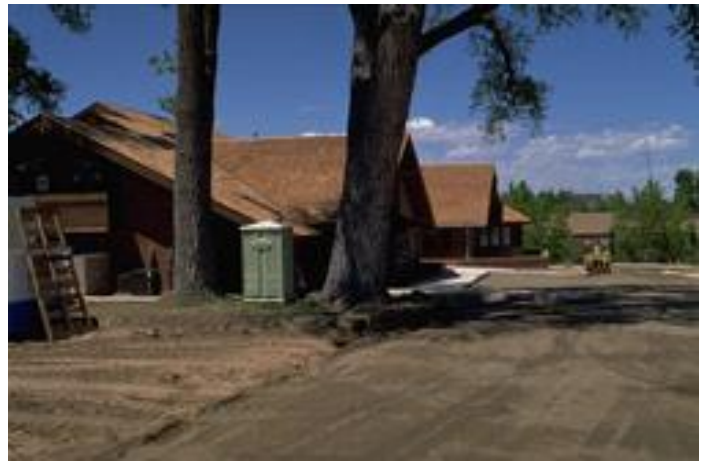
Figure 4: Surface grading severs many roots.
