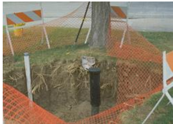
Figure 1: Roots lie in the upper 60 cm (24 inches) of soil and are easily damaged.
