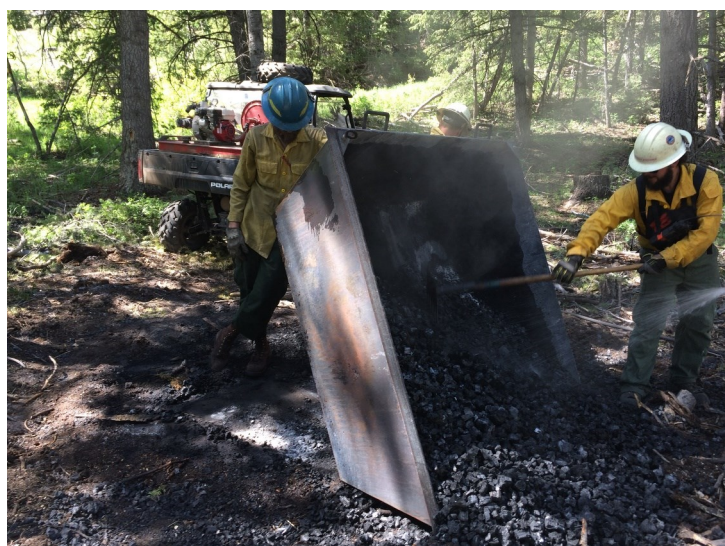
Figure 14. Quenching biochar in a series of steps.
